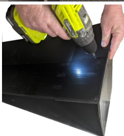
4. Assemble height adjusted Modular Wall extension section and secure with self tapping screw
