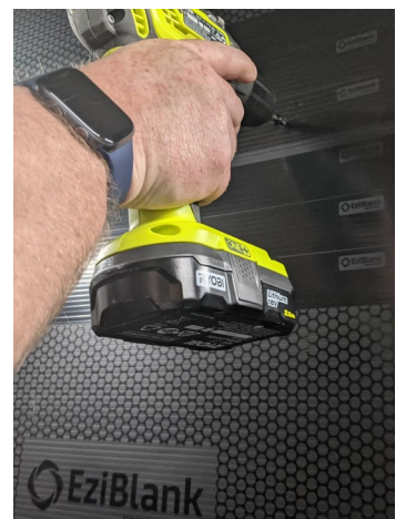
6. Secure new section with self tapping screw
