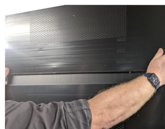
5. Position newly completed Mod Wall section on top of existing Wall structure
